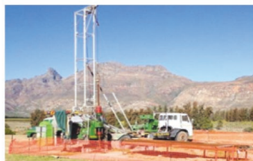
Drill rig used in April 2012 on site
